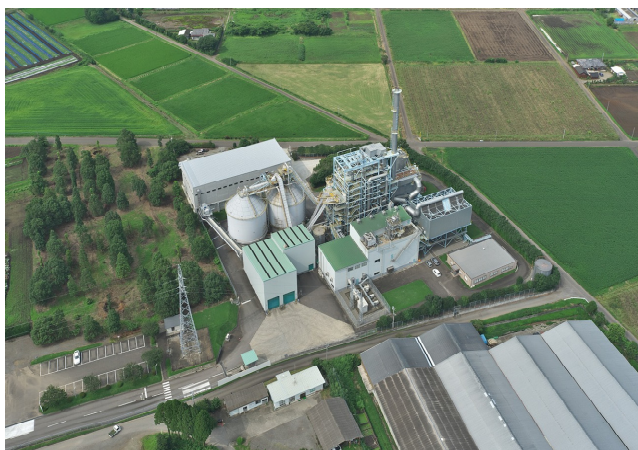
Fig. 9 Power plant for generating electricity by incinerating broiler chicken manure. Photograph courtesy of K. Yano (Miyazaki Biomass Recycle Co.).
